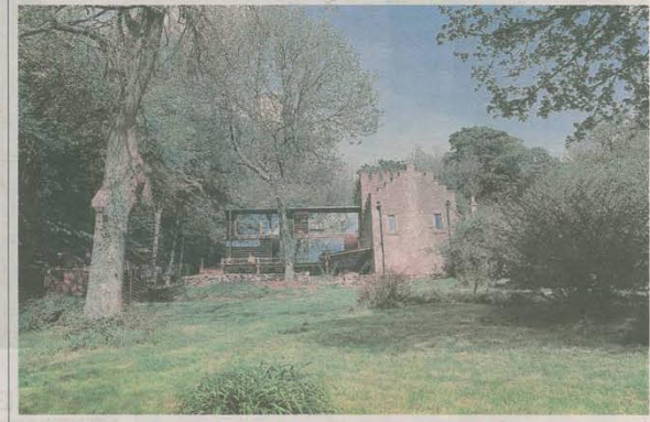
With a lightweight, see-through extension on the left and solid stone walls on the right, the house is a study in contrasts
