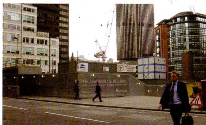
British Land's Leadenhall site in the City of London.
