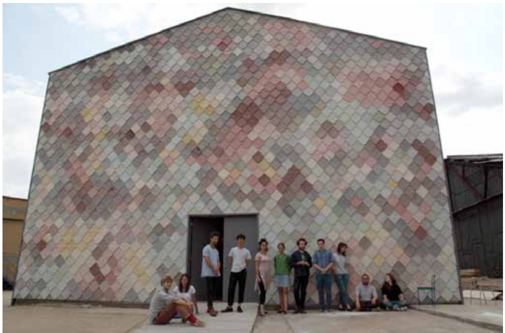
Assemble at its self-built Yardhouse in Hackney Wick, complete with coloured concrete shingles made on site.
