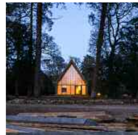
Above, right Mess room interior views; south-facing elevation in timber and polycarbonate (phs: AM)
