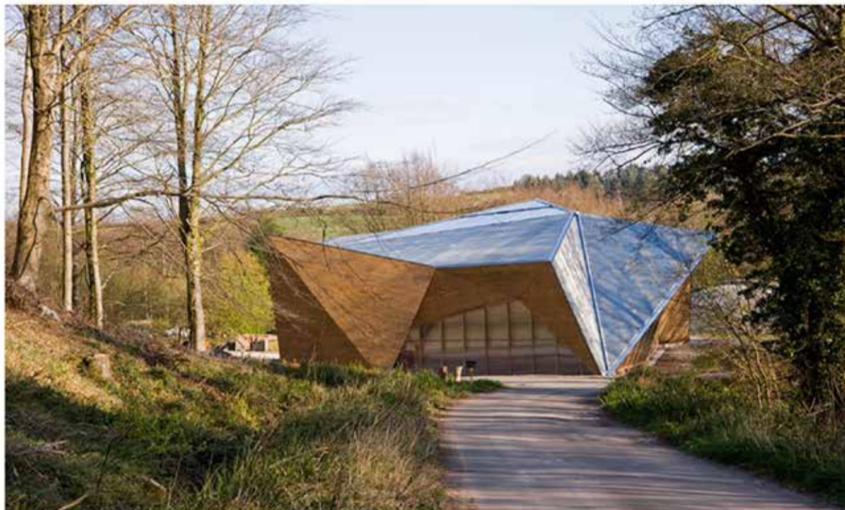
the angular form is located in hooke park, made from a variety of local timber image © valerie bennett (also first image)
