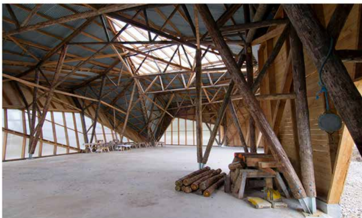
a series of trusses developed with engineers uses felled natural tree trunks as research into the use of irregular planks for complex shapes image © valerie bennett
