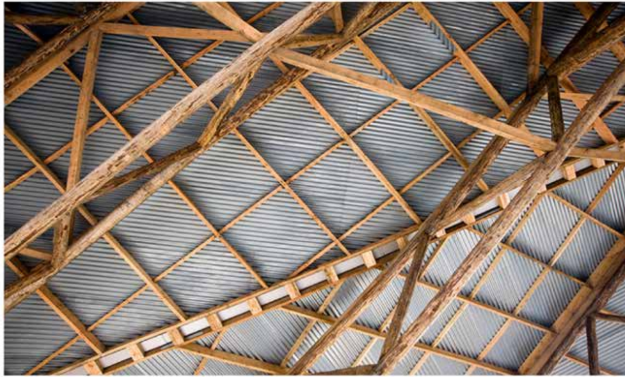
corrugated sheets provide a low maintenance roofing material capable of cladding the irregular form image © valerie bennett corrugated sheets provide a low maintenance roofing material capable of cladding the irregular form image © valerie bennett
