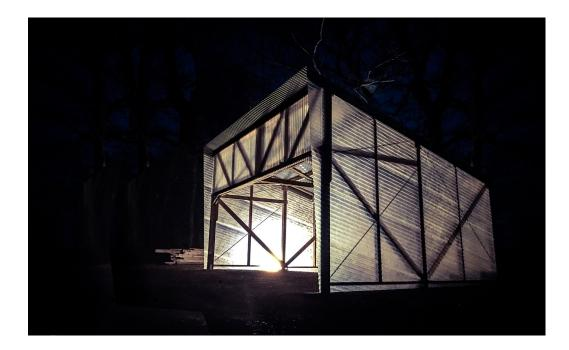
This ethereal-looking prototyping workshop in Wiltshire was designed by Invisible Studio. With its pared-down, spare aesthetic, its constructional efficiency reflects their approach to design, exploring contingency in the construction process – and using minimal drawings.
