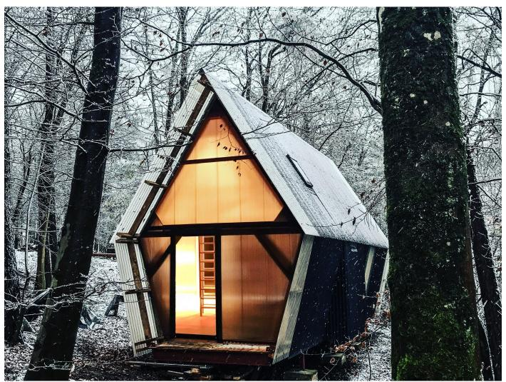
This self-built, relocatable prototype was built from construction waste and locally grown unseasoned timber
