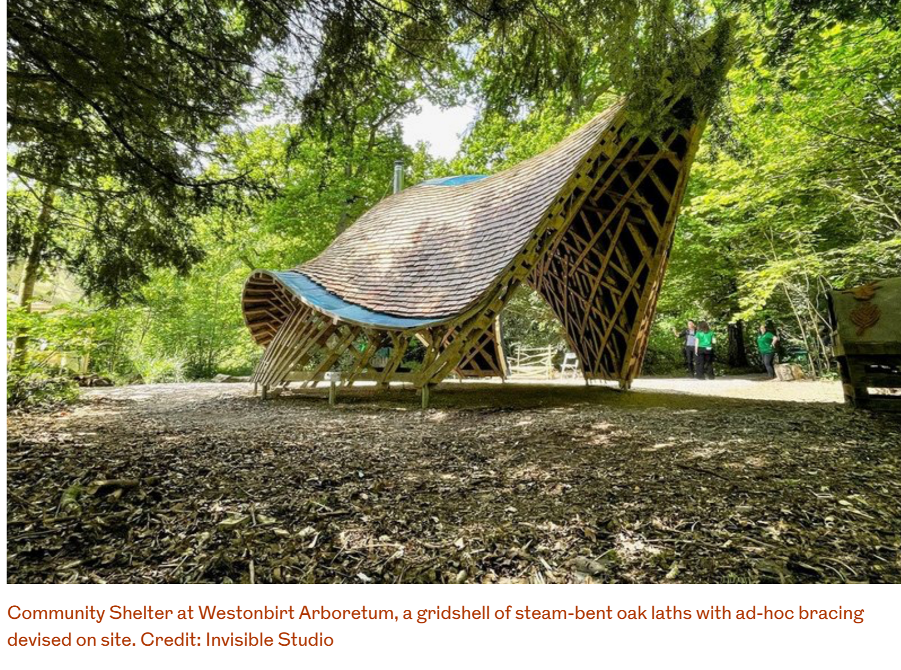
Community Shelter at Westonbirt Arboretum, a gridshell of steam-bent oak laths with ad-hoc bracing devised on site. Credit: Invisible Studio
